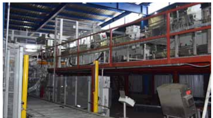
Work continues on the Palletizer and De-Palletizer in the Beer Plant
